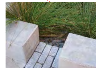
Runnels channel water across the site and plants filter the water before it enters a cistern for re-use as irrigation or toilet flushing
