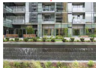
A bio-swale and a recycled water feature serve as a buffer between semi-public and private open spaces without the use of fences.
