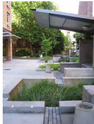
Runnels channel water across the site and plants filter the water before it enters a cistern for re-use as irrigation or toilet flushing
