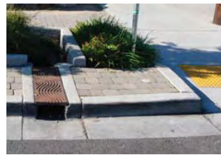
Flow-through planters along streets reduce peak flows by holding water. The storm sewer system serves as an overflow.
