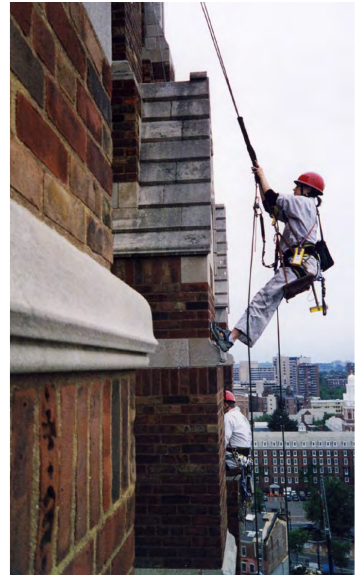
Yale graduate dormitory inspection
