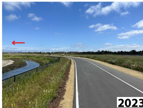
Photographs C. Digital and digitized photographs of the levee and trail taken east of Sea Cloud Park along Belmont Slough looking northeast in 1990, 2019, and 2023. The 1990 photograph provides a close approximation of the original master plan design while the 2019 image shows the improvements made in 1991 including an additional earthen berm, trail widening, and a habitat exclusion fence. The 2023 image shows a raised and widened trail with the habitat fence relocated to the bottom of the slope to increase visual access. A radio tower is marked by an arrow in each photograph to provide a relative location. The 1990 digitized image is part of the BCDC permit 1991.016.00 record file. (BCDC, 1990; A.Gaffney, 2019, 2023)
