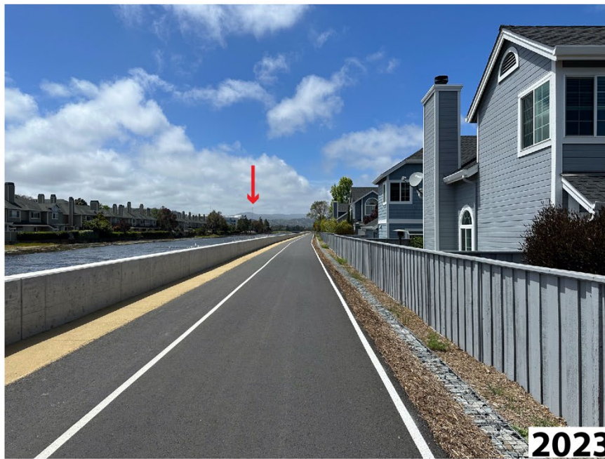
Photographs E. Digital photographs of the levee and trail taken along O’Neill Slough west of Port Royal Park looking west in 2018 and 2023. A radio tower is marked by an arrow in each photograph to provide a relative location. The two-foot-tall floodwall pictured in the 2018 photograph was installed in the 1990s. The 2023 photograph shows the grade of the trail has been elevated approximately two feet, with a widened area for the trail, placing the 30-inch-tall floodwall closer to the water. (A.Gaffney, 2018, 2023)
