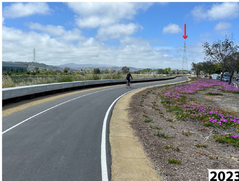
Photographs D. Digital photographs of the levee and trail taken along Belmont Slough and Timberhead Lane looking southwest in 2019 and 2023. An electrical transmission tower is marked by an arrow in each photograph to provide a relative location. The low earthen berm pictured in the 2019 photograph was installed in the 1990s. The 2023 photograph shows the trail has been widened and kept at the same elevation, placing the 30-inch-tall floodwall closer to the water. (A.Gaffney, 2019, 2023)
