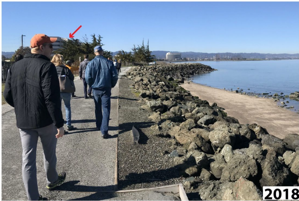
Photographs 3. Digital and digitized photographs of the levee and trail taken north of the San Mateo Bridge looking southwest in 1990 and 2018. The 1990 photograph provides a close approximation of the original master plan design while the 2018 image shows the improvements made in 1991 including additional riprap and trail widening. An adjacent building is marked by an arrow in each photograph to provide a relative location. Construction of this section of the levee and trail was not yet complete on July 31, 2023, but will be documented when it's open to the public in August 2023. The 1990 digitized image is part of the BCDC permit 1991.016.00 record file. (BCDC, 1990; A.Gaffney, 2018)
