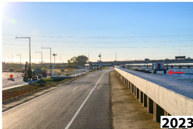
Photographs A. Digital and digitized photographs of the levee and trail taken near Beach Park Boulevard along the San Francisco Bay north of Egret Street looking northwest in 1990, 2019, and 2023. The 1990 photograph provides a close approximation of the original master plan design while the 2019 image shows the improvements made in 1991 including additional riprap and trail widening. The 2023 image shows a reconstructed access point, a raised and widened trail, and a seawall. The San Francisco Airport beacon station is marked by an arrow in each photograph to provide a relative location with the San Mateo bridge in the background. The 1991 digitized image is part of the BCDC permit 1991.016.00 record file. (BCDC, 1990; A.Gaffney, 2019, 2023)
