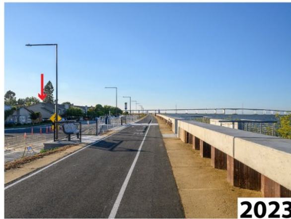
Photographs B. Digital and digitized photographs of the levee and trail taken near Beach Park Boulevard along the San Francisco Bay south of Marlin Avenue looking northwest in 1990, 2018, and 2023. The 1990 photograph provides a close approximation of the original master plan design while the 2018 image shows the improvements made in 1991 including additional earthen berm and trail widening. The 2023 image shows a reconstructed access point, a raised and widened trail, and a seawall with a waterside overlook. A house is marked by an arrow in each photograph to provide a relative location. The 1990 digitized image is part of the BCDC permit 1991.016.00 record file. (BCDC, 1990; A.Gaffney, 2018, 2023)
