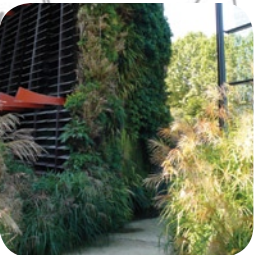
Vegetated roofs and walls capture rainwater and reduce runoff.
