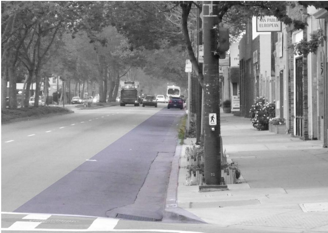
Parking lane isolated in color. No difference in paving exists for the parking lane, only the gutter.
