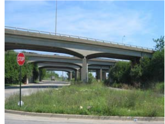
Existing cut-through at East Witherspoon looking north.
