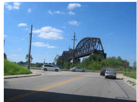
Existing cut-through at East Witherspoon and River Road.
