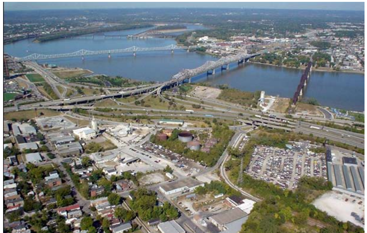
Image of existing site Source: Immediate Needs Report
